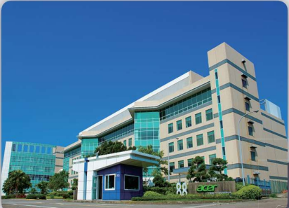
Data Center-Tech Industry
