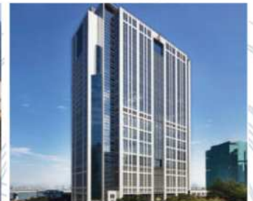
Customs Headquarters Building, Hong Kong
