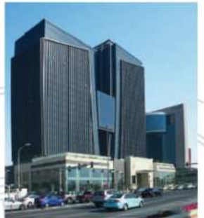
Al Shoumoukh Tower, Qatar
