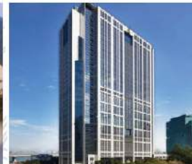
Customs Headquarters Building, Hong Kong
