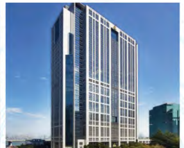
Customs Headquarters Building, Hong Kong
