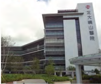
Lantau Hospital, Hong Kong
